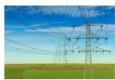
Lattice towers for transmission lines Up to 1,200kV; over 0.50mn MT supplied since 1998
